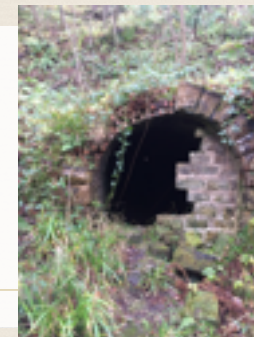
Former narrow gauge railway tunnel
